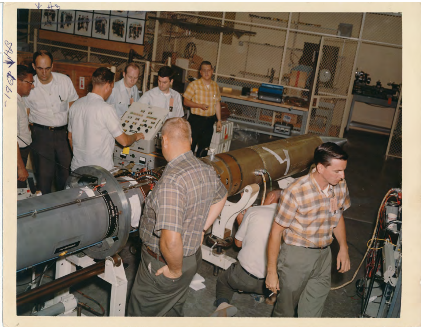
Horizontal test of the first NASA/MIT Sounding Rocket 4.190, White Sands Missile Range, June 29, 1967. Hale Bradt (far left facing this way), Edward Boughan, Saul Rappaport, and Don Fairbrother(?) (left to right facing this way in center rear), Joseph Morris(?) (facing away in foreground). (NASA Photo)
